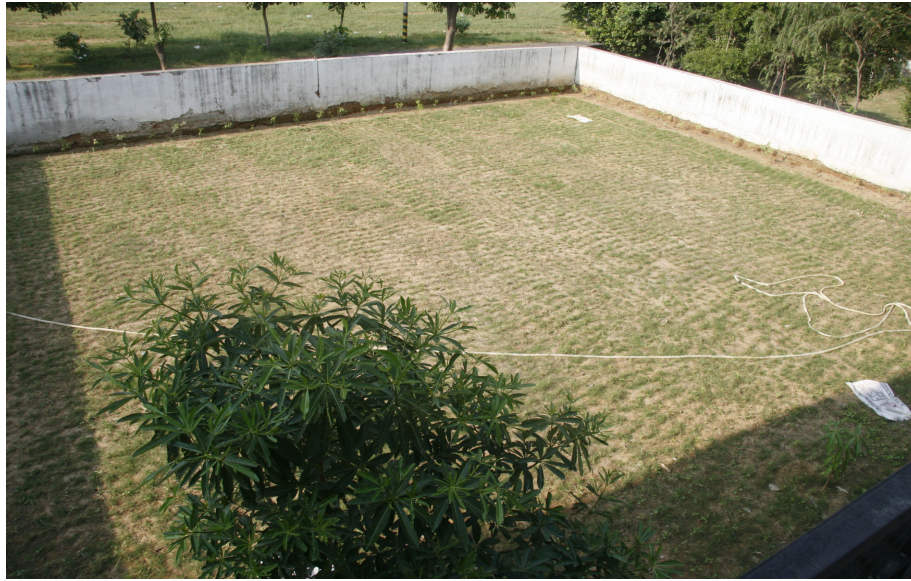
Preparation of backyard in progress
